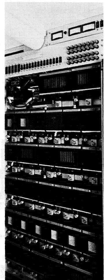
All equipment easily accessible
